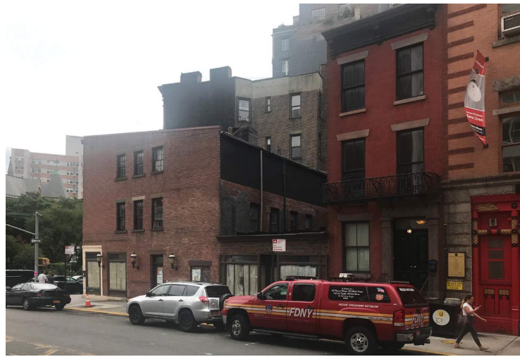
EXISTING WEST 10TH STREET FACADE (2019)
